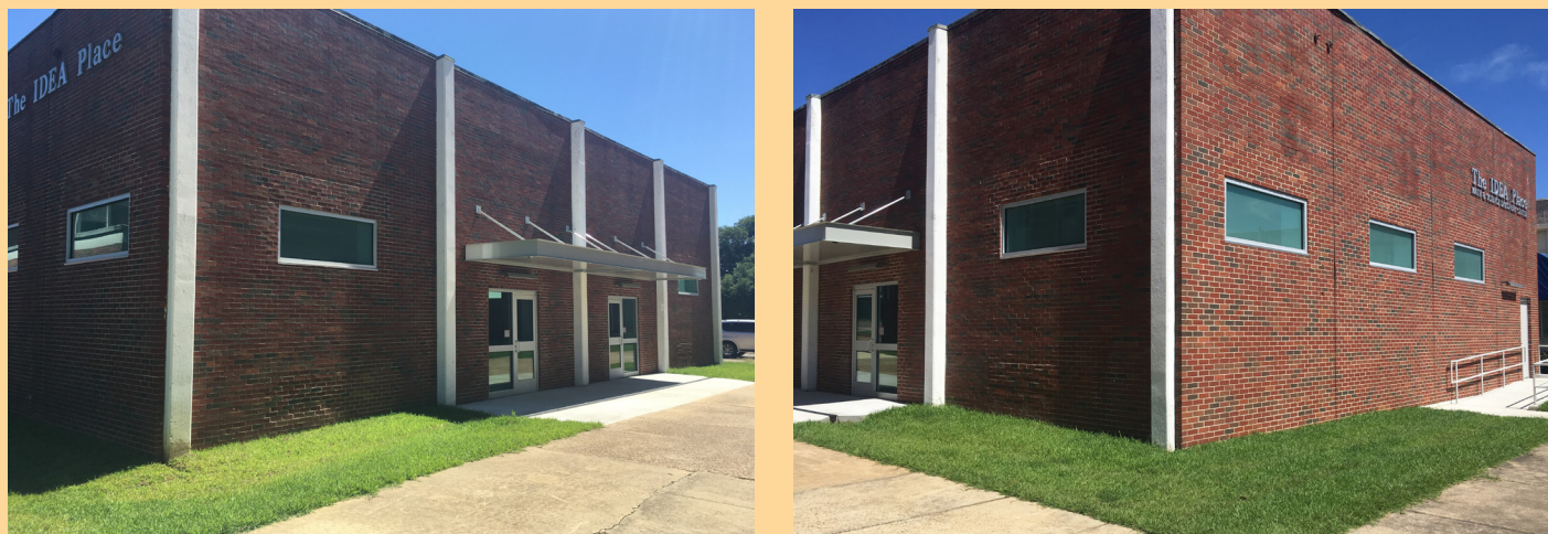
Figure 1: The (a) south (main) entrance and (b) southeast corner of the IDEA Place show the void landscape after the recent renovation. (Photos by Kelsey Shoemaker. June 10, 2020.)
